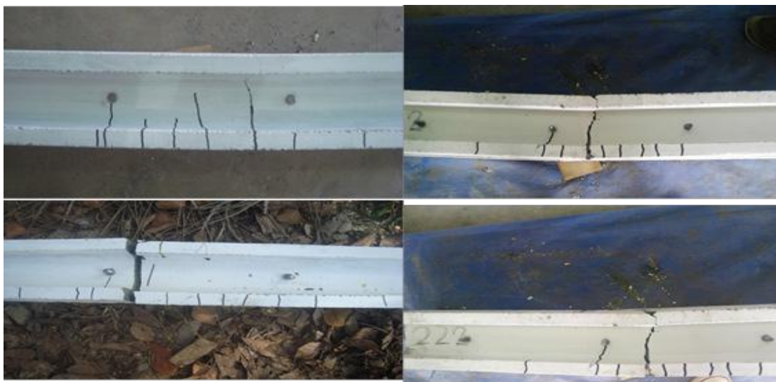
Figure 8. Actual Cracking Pattern of the Beam at Failure
